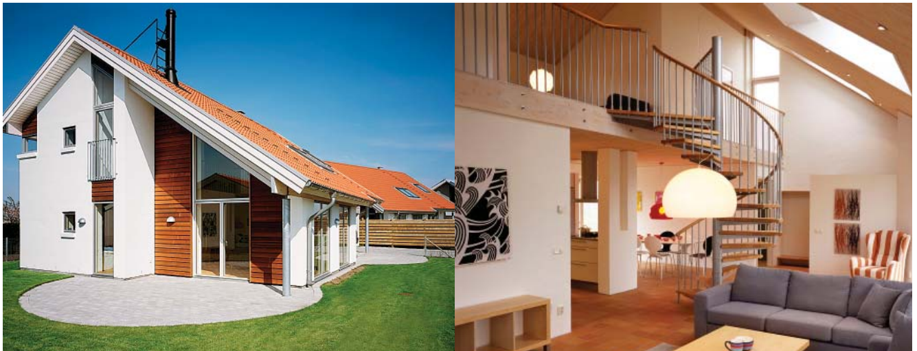
Uniqhus offers Sweden's first environmentally labeled housing. Skanska's sustainable housing concept received a Swan-labeling license during 2005. Uniqhus was environmentally certified after an examination by SIS Ecolabelling AB. Using environmentally friendly materials and construction methods combined with low energy consumption, Uniqhus has a low life-cycle cost. The first Swan-labeled Uniqhus homes were built in Malmö, with a February 2006 move-in date.
