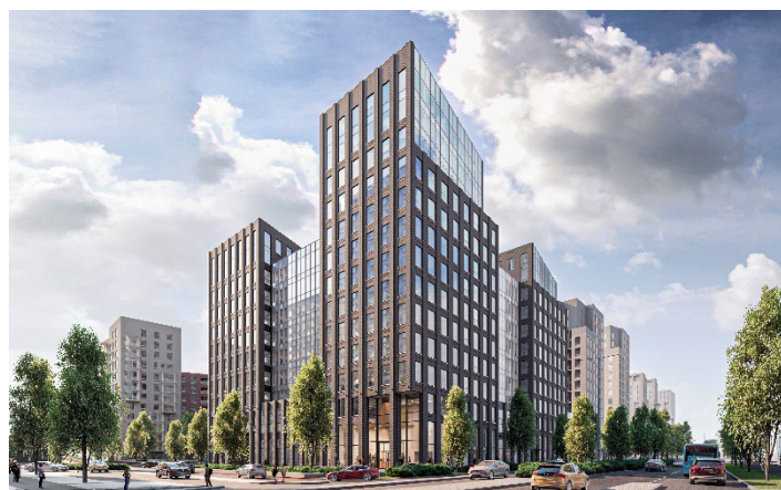
Investment: office project Firdo, Helsinki, Finland
