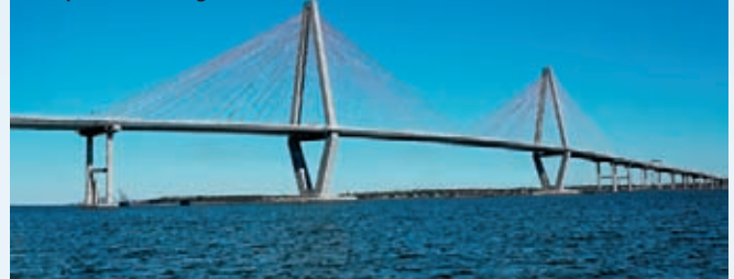
Cooper River Bridge
